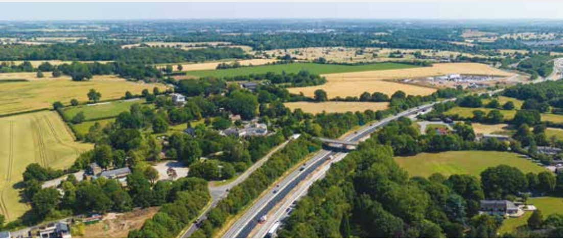
A12, Essex Reconstruction Works
