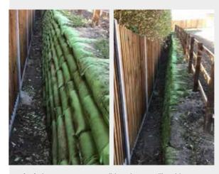
At Acle, a geo-grow wall has been utilised in place of a traditional brick retaining wall. The vegetated wall system is made up of geotextile
