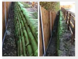
At Acle, a geo-grow wall has been utilised in place of a traditional brick retaining wall. The vegetated wall system is made up of geotextile bags, constructed into a permanent wall, it requires minimal equipment and labour and acts as a sustainable and visually appealing solution. Attracting biodiversity to the area, contributing to carbon saving, reducing surface water runoff and providing a more natural aesthetic.
